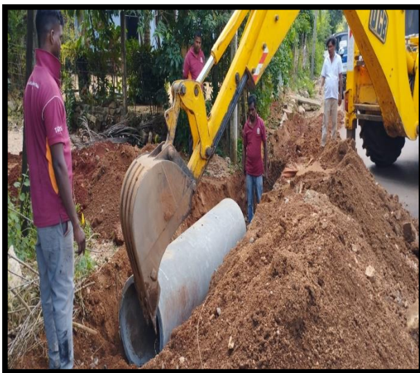
Laying Hume Pipes lional Fernando mawatha andankulam
