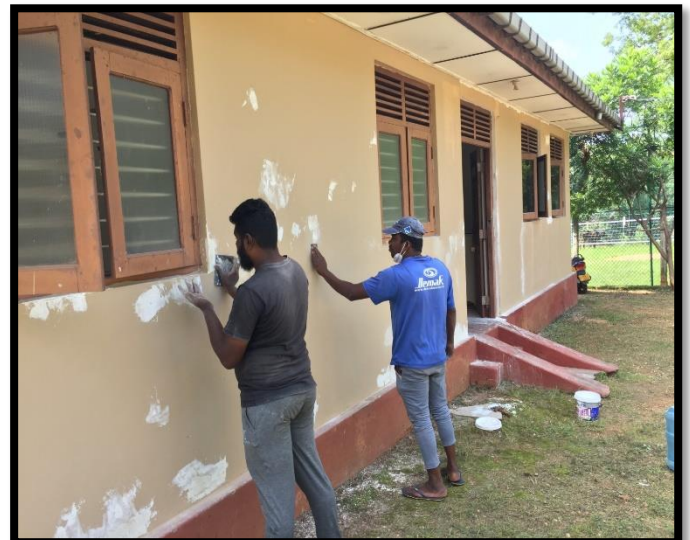
Singapura community Centre Building Repairing Work
