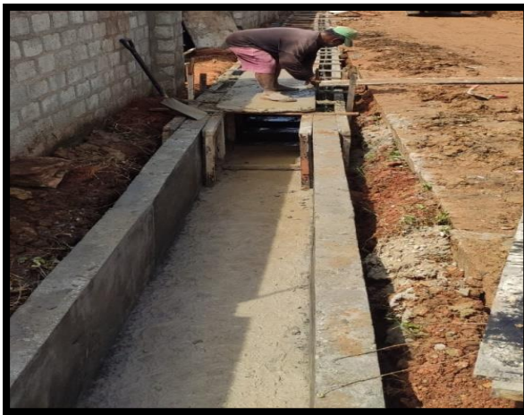
Completion of Concrete Drainage at Sumethangarapura Internal Road, Sumethangarapura, Trincomalee.
