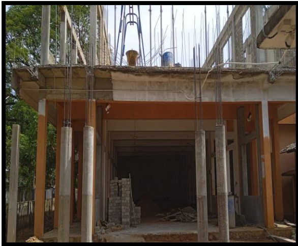
Completion of Multi Purpose Building at Puliyankulam
